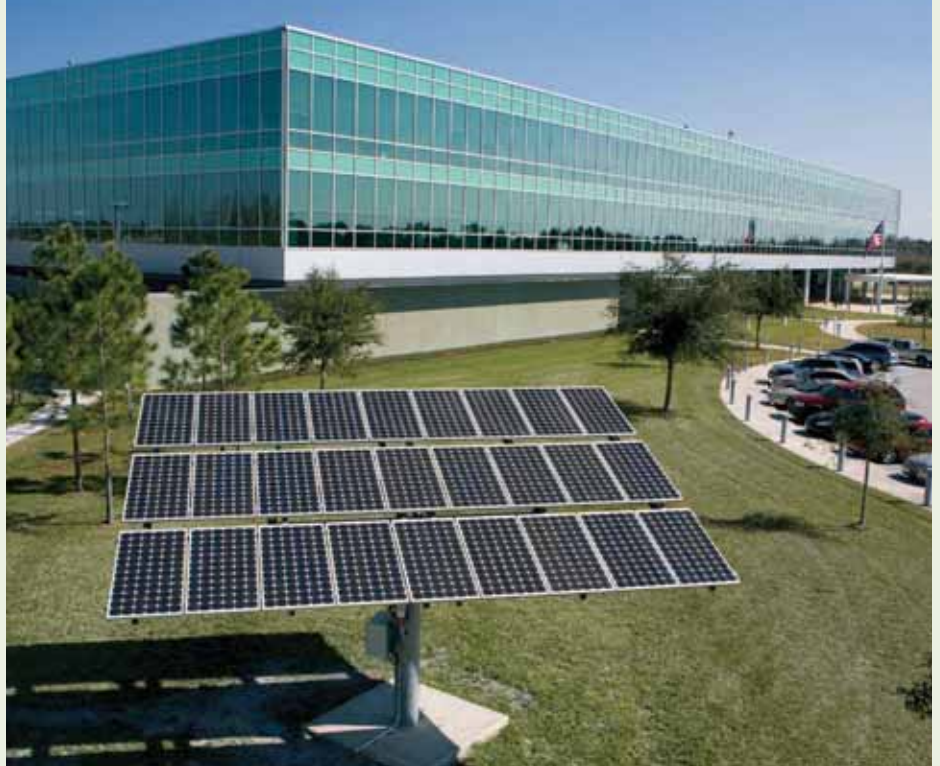
Solar power is an ongoing priority for Publix. The company currently has four different locations that benefit from solar energy.
